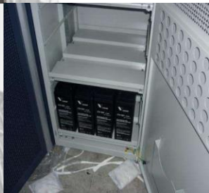
EQUIPMENT INSTALLATION (DMDW, METRO-E)
