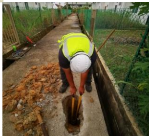
CONCRETE POLE INSTALLATION
