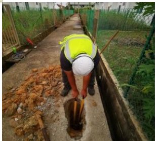
CONCRETE POLE INSTALLATION
